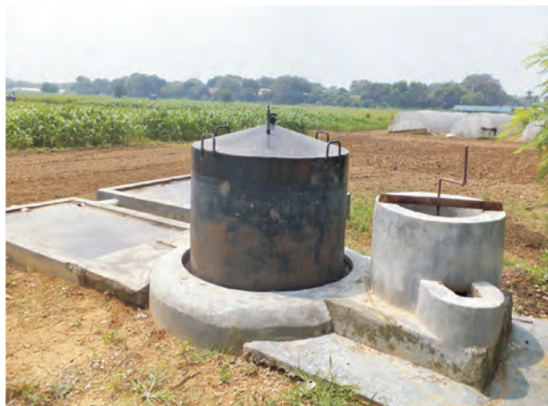
Fig. 18: Design of biogas plant used
