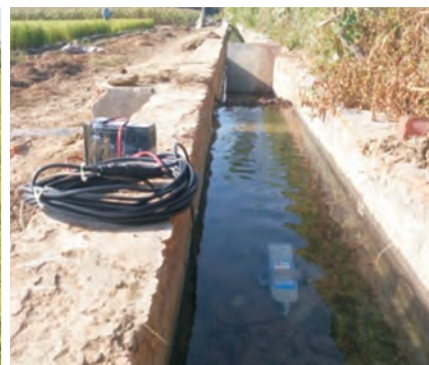
Water measurement using starflow meter
