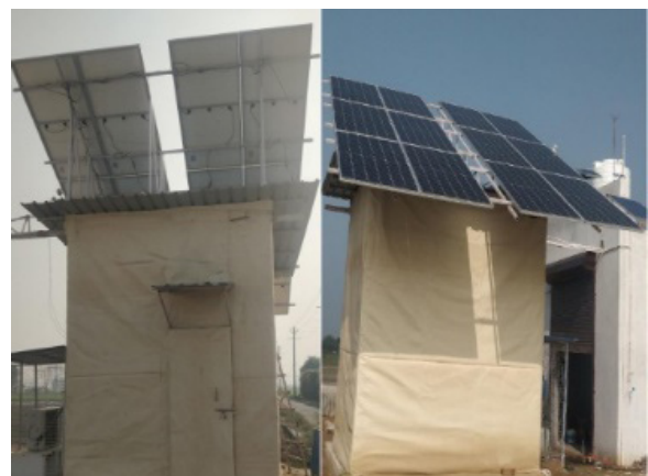
Pusa Farm SunFridge at village Cullakpur
